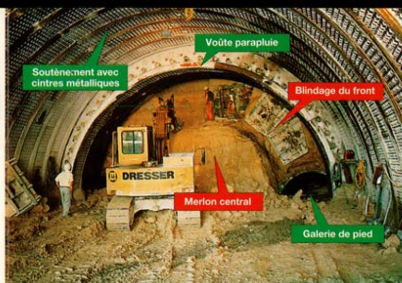
Excavation (Document Bureau Ing. Bourquin, Neuchâtel)
